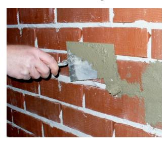
On porous concrete, Autoclaved Aerated Concrete, or on soft brick, a sound plaster made of KÖSTER Repair Mortar must be applied.
