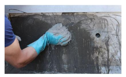
The "ball" is firmly pressed onto the leak. After a few seconds the leak should be stopped. We suggest using smooth rubber gloves when processing KÖSTER KD 2 Blitz Powder.
