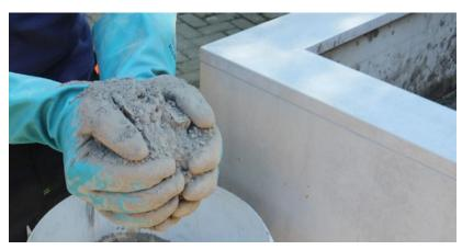
In areas with stronger leaks including an active water spout, a larger amount of KÖSTER KD 2 Blitz Powder is pressed into a ball between both hands, compressing as much air out as possible.
