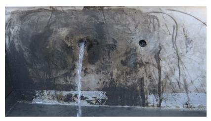
Depending on the intensity of the active leak, a sufficient amount of dry powder is applied by hand directly to the active leak without adding any extra water. In case of small active leaks where water slowly drips from the wall, the powder is rubbed firmly onto the surface until the leakage is stopped.
