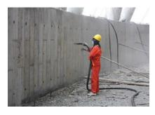
**Sandblasting** or **shotblasting** Suitable for creating a CSP-2 to CSP-8.
