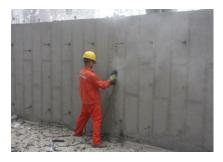
**Grinding**Suitable for creating a CSP-1 to CSP-3.
